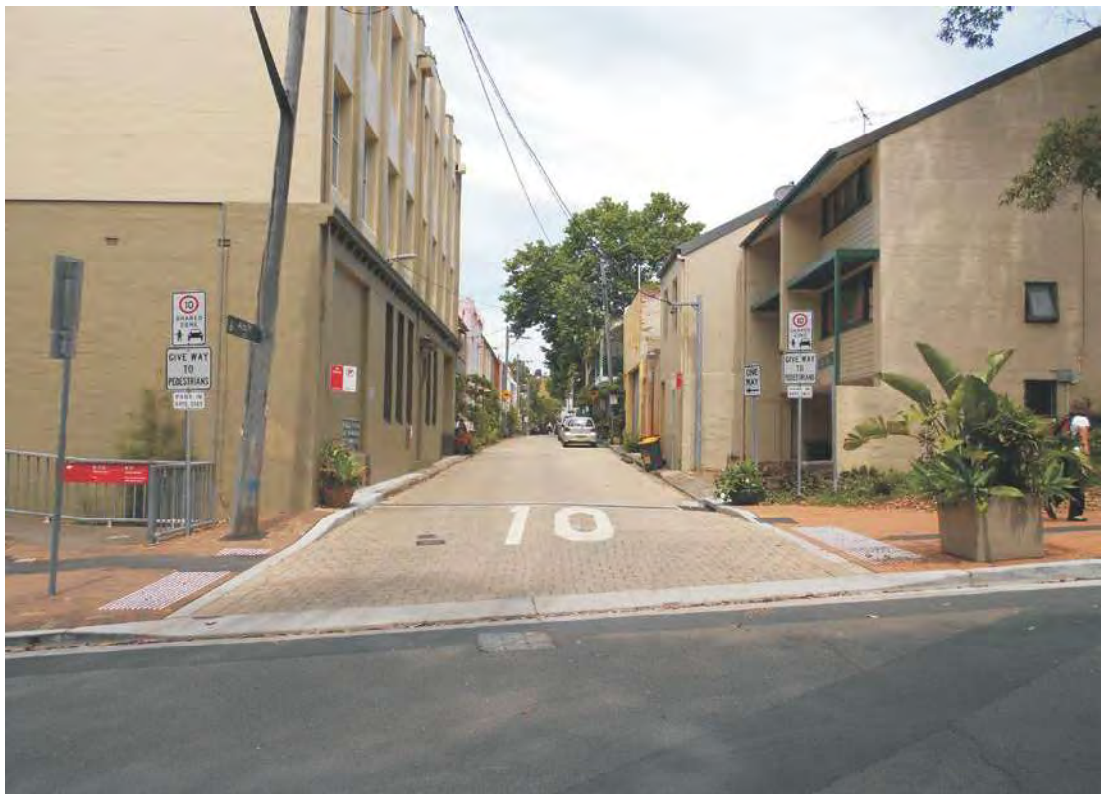
Figure 1. Photo and diagram of a Category 1 shared zone showing regulatory signage, typical layout and treatments. [Note: The No Entry sign is site specific] The photo may have been modified to demonstrate essential elements.
